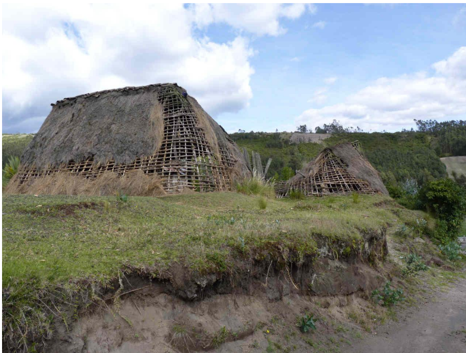
Partially dilapidated traditional farm houses revealing the construction principle
